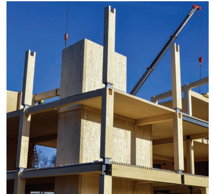
Glulam laminated wood constitutes beams and columns for the UMass, Amherst, Olver Building. photo © by Alex Schreyer
