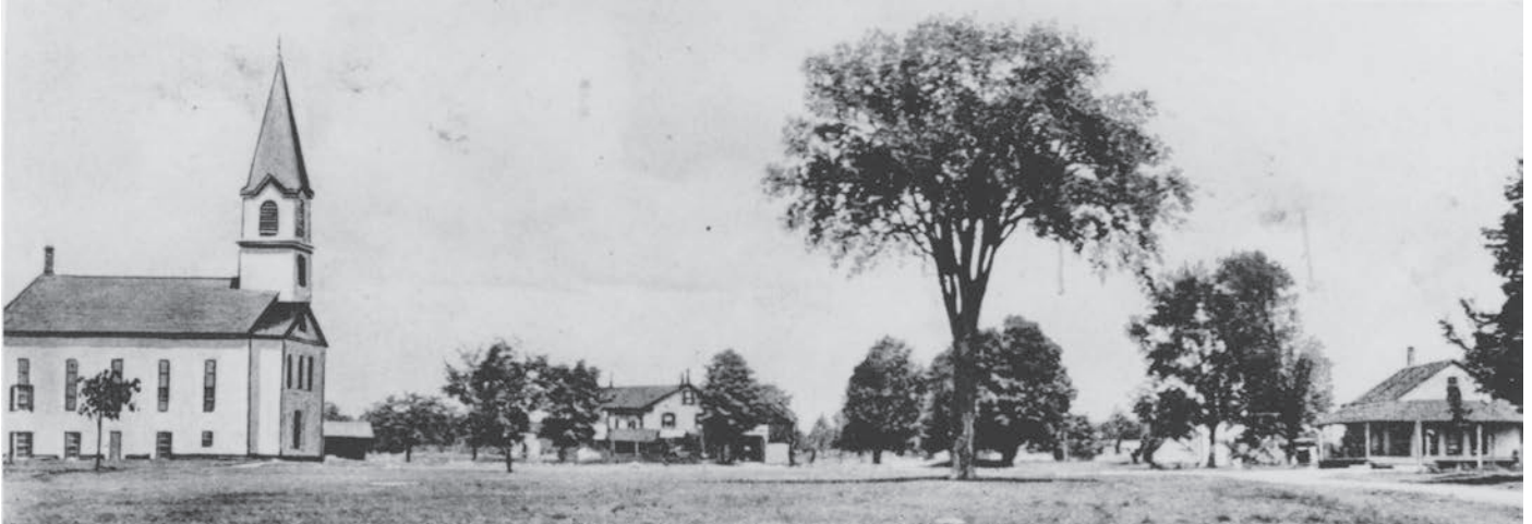
Before the reservoir, Greenwich Congregational Church, Walker's Hall Store, and Farmers' Hall bordered the town common.
