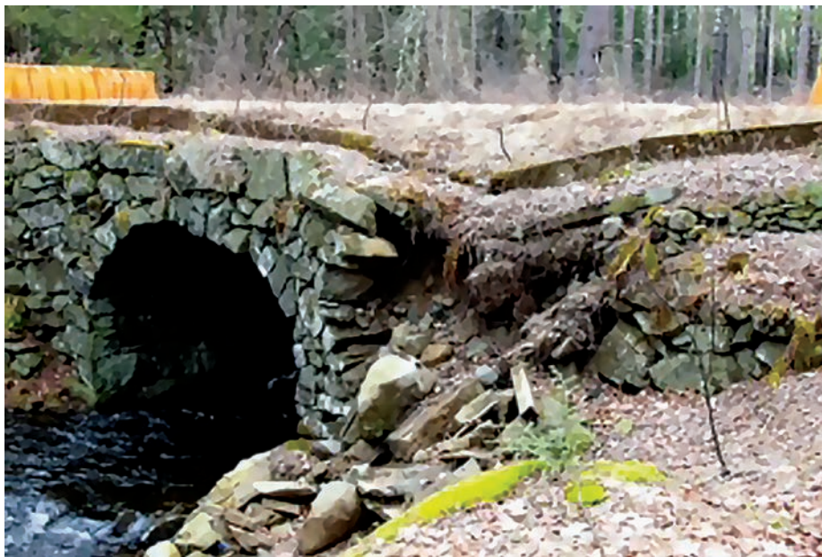
Not far from Quabbin Reservoir Gate 30, Keystone Bridge requires repair, as shown at right of the arched bridge.
