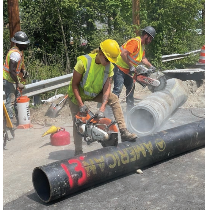
Rachel O'Dell of Barre sizes a culvert pipe. photo courtesy of Rachel O'Dell
