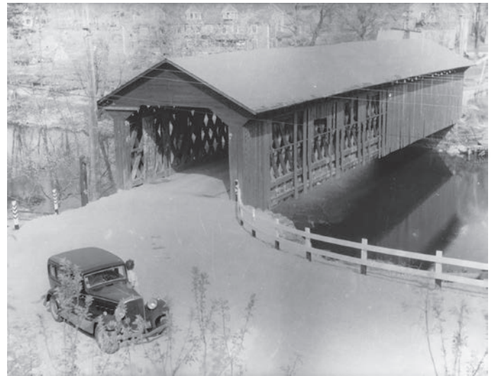
The Ware-Gilbertville Bridge, the only remaining covered bridge in central Massachusetts, from a 1939 image by William Maxant, who photographed many of New England's covered spans during the mid twentieth century. Exposed frame and missing boards show on Ware's side of the structure.
