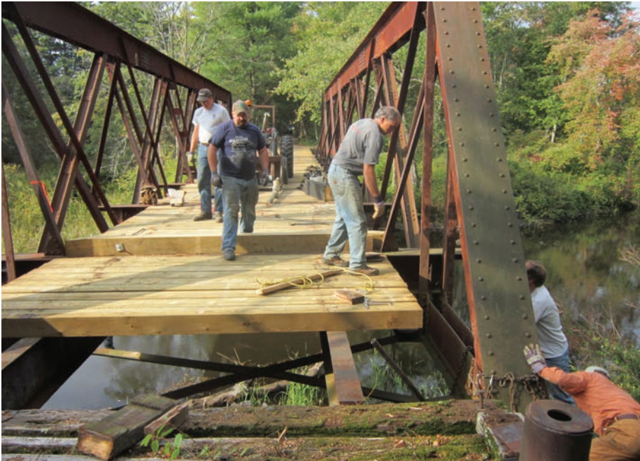
Workers rehabilitate an old railroad trestle to accommodate recreational users in a new rail trail sponsored by East Quabbin Land Trust along the Ware River. photo © by Cynthia Henshaw
