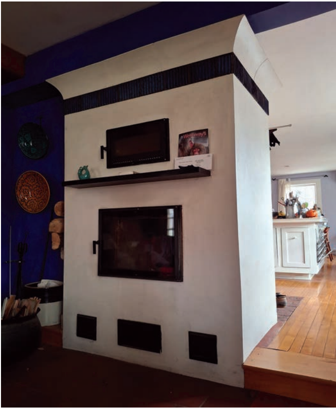
A Finnish masonry stove efficiently burns wood at high temperature to heat a regional residence.
