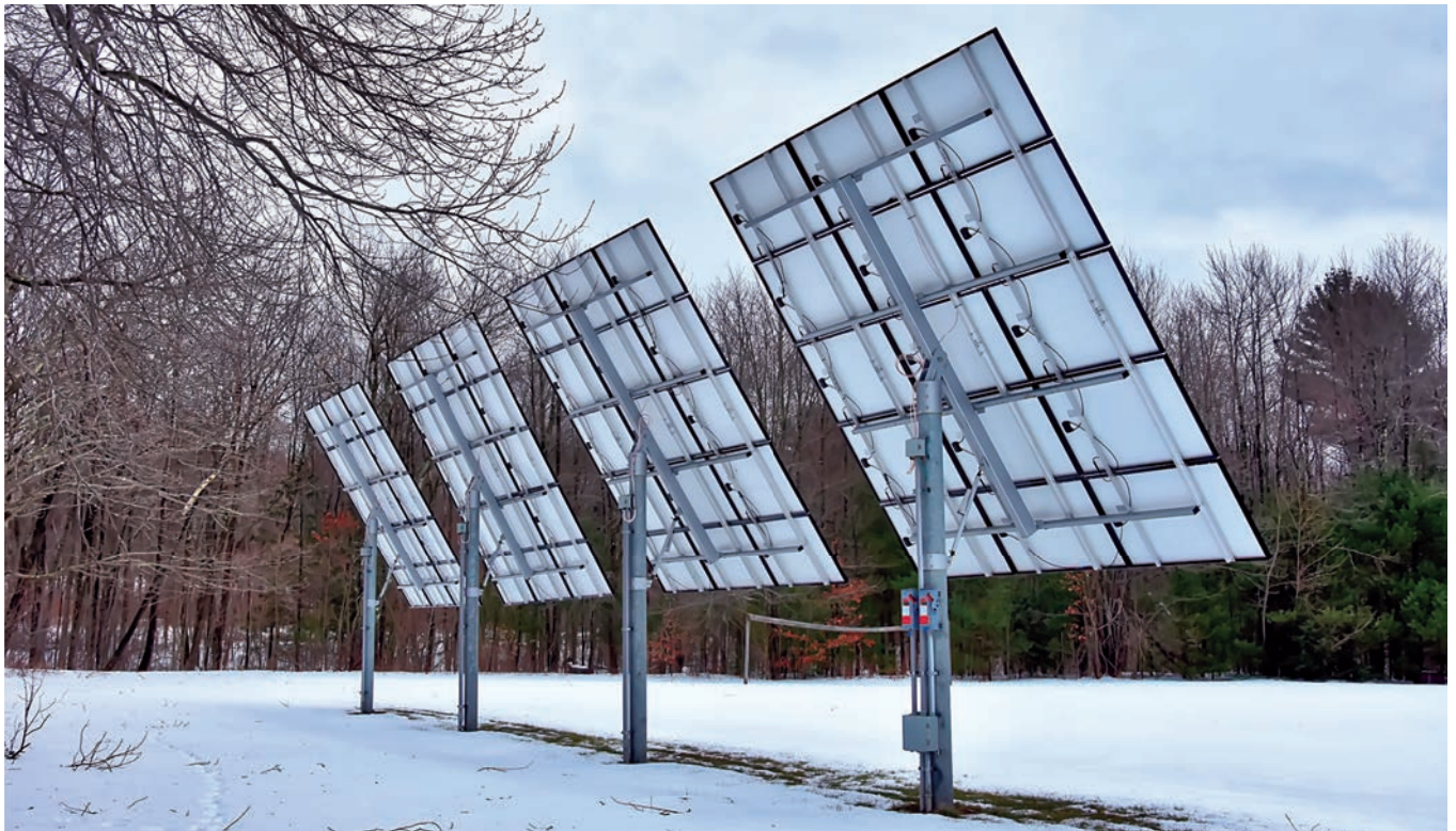
Green Communities funds provided the Shutesbury Fire Department with a thirteen-kilowatt pole-mounted photovoltaic (pvc) solar installation to provide electrical energy. photo © by Mitchell R. Grosky
